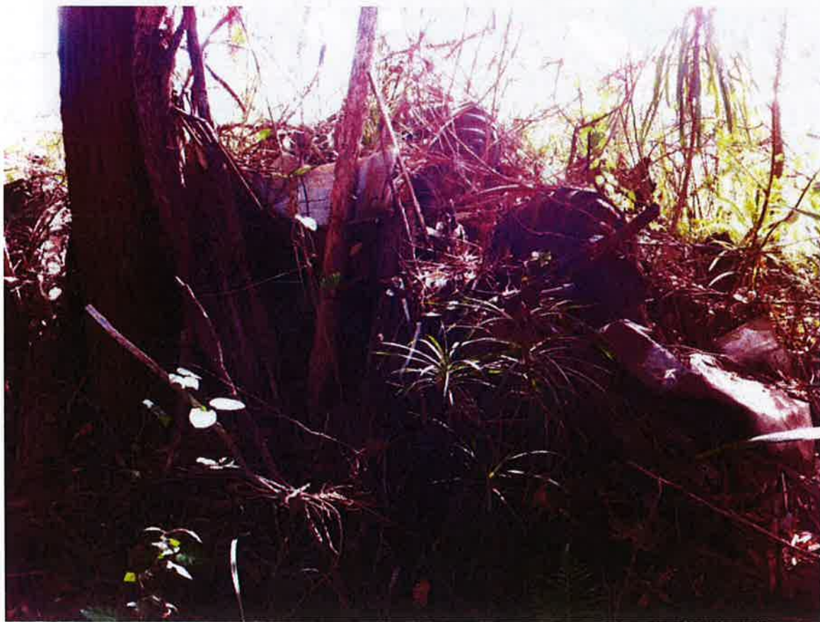
Figure 3. Building waste in zone 1
